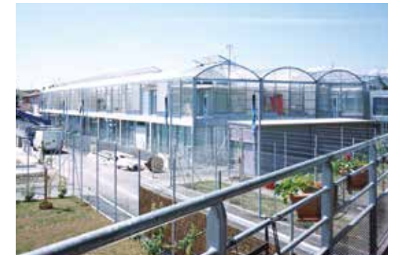
Rental units, Lacaton & Vassal.
