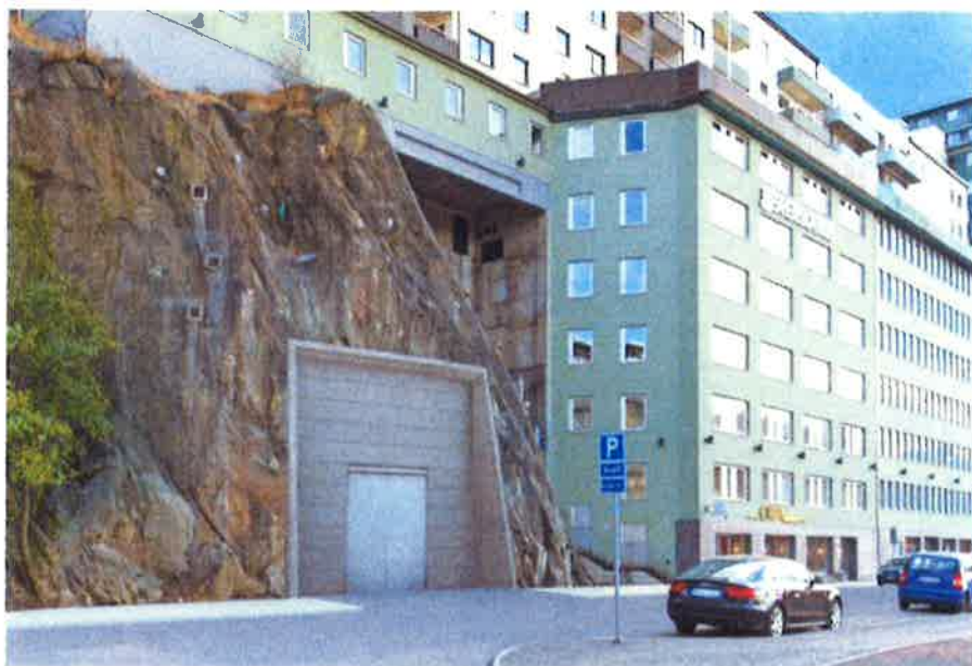
Servicetunnel- mynning Stora Badhus- gatan
