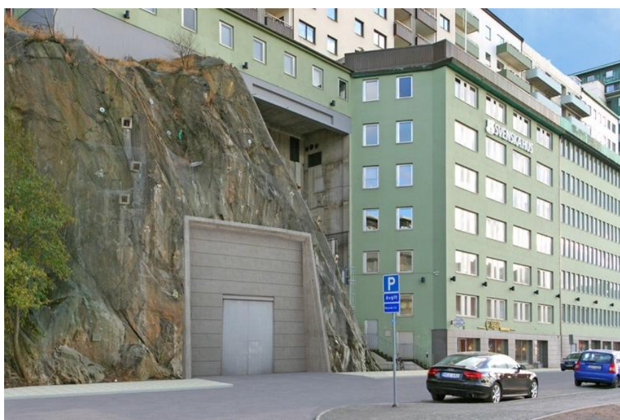
Servicetunnel- mynning Stora Badhus- gatan
