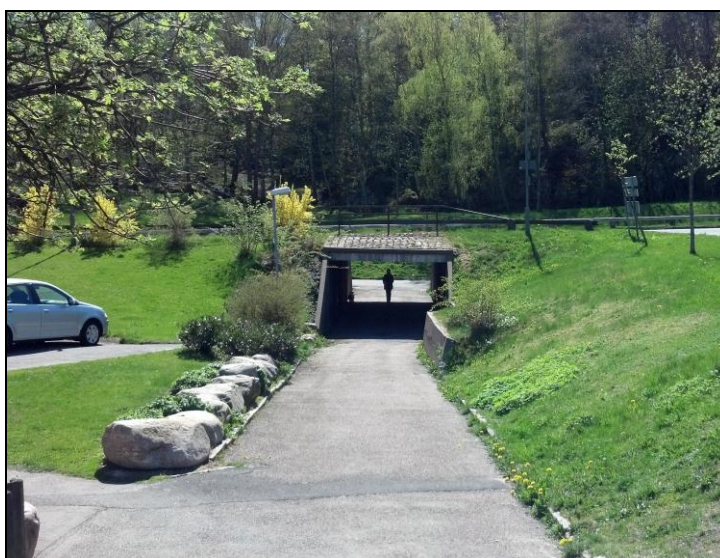
Figur 5. Viadukt under Opalgatan
