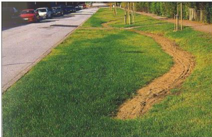
Figur 10 Svackdike (Ref: Peter Stahre)
