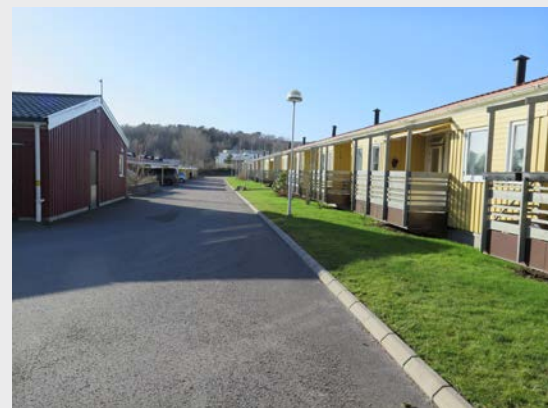
Kv Panelen: Toftåsens radhus
