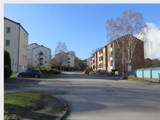
Kv Brandmuren, Cementen
