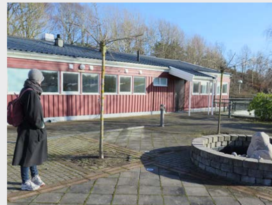
Kv Panelen: Toftåsens radhus
