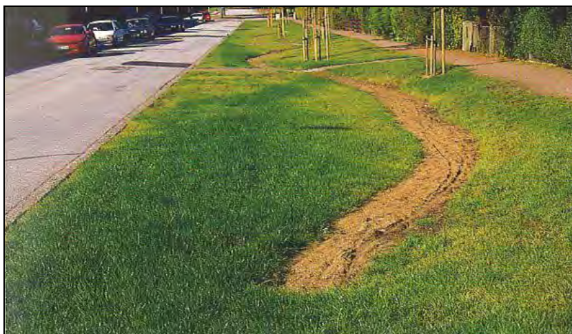
Figur 11. Svackdike (Ref. Peter Stahre)
