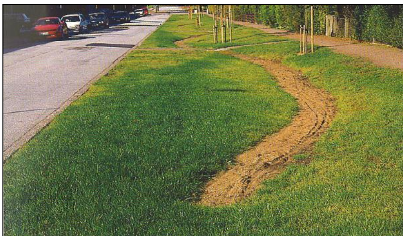
Figur 11. Svackdike (Ref. Peter Stahre)
